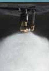
The average Victaulic Vortex droplet size is less than 10 microns, and the minimal amount of water released per emitter—as little as one gallon per minute—virtually eliminates any wetting in a space.
