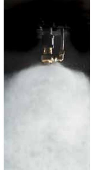
The unique swirling pattern quickly fills the hazard space and attacks the fire, overcoming aerodynamic forces that typically decelerate and diffuse water droplets making them ineffective.
